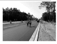
Log Creek, eight stormwater ponds, curb and gutter, drainage, earthwork, grading, and paving. This project included four large box culverts and substantial geotechnical work including geo-grid stabilized fill and embankment surcharge.
