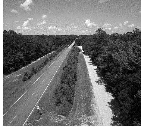
As a result of the widening, the new roadway front slopes will be constructed. The typical 1:6 slope will be maintained throughout the project except for geometric constraint areas such as locations where there is not enough right of way, or high fill areas or culverts to tie into. Front slopes are a major safety aspect of any roadway, and our inspectors will make sure that the front slopes meet the required template within the entire project.
