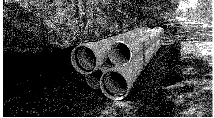
North Street Transmission Main & Bluffton Parkway Transmission Main, Beaufort-Jasper Water & Sewer Authority, Okatie SC: Through a collaborative design process, Barge rerouted the proposed pipeline saving the client approximately $1.6M in overall costs.
