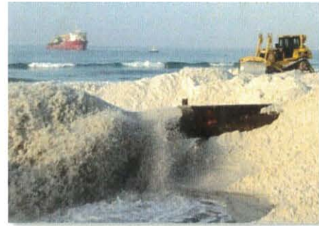
Destin/Walton Beach Restoration
