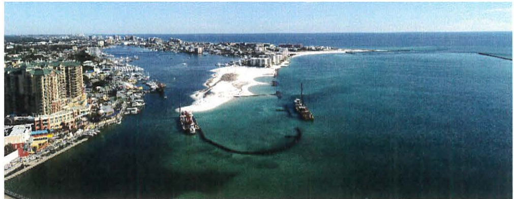
Norriego Point During Construction (December 2017)
