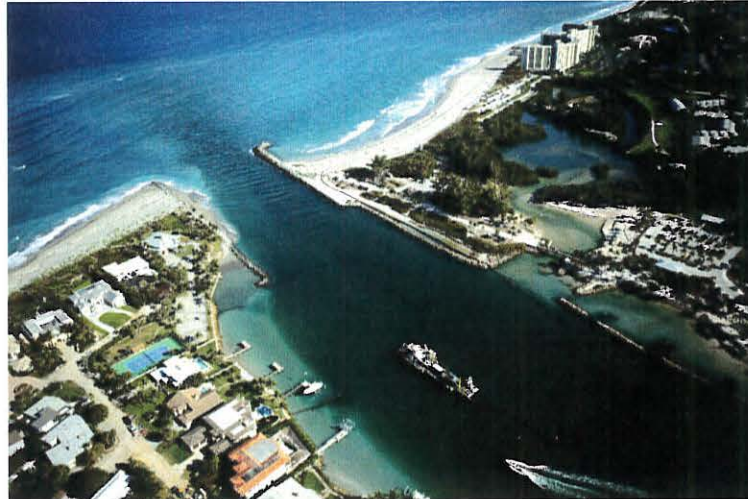
Beach construction during Jupiter Inlet sand trap dredging
