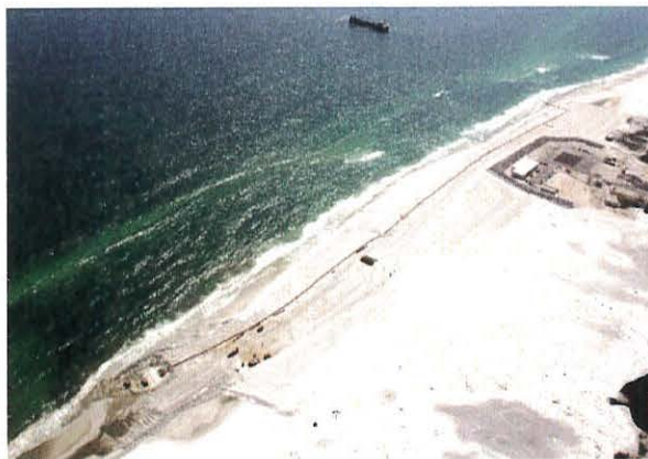
Eglin AFB Site A-3 during construction
