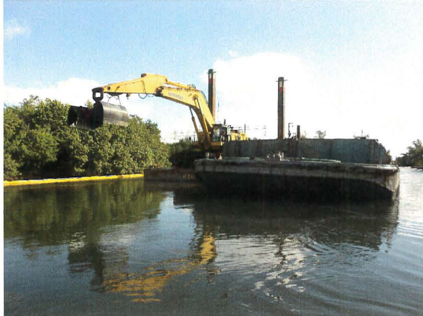
Mechanical Dredge within the Dania Cutoff Canal
