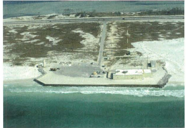
Eglin AFB Site A-3 pre-construction condition
