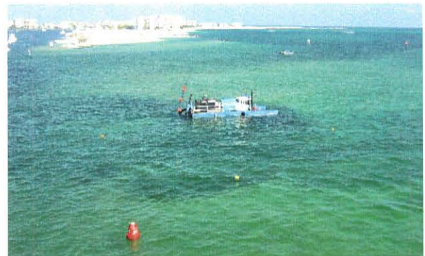
Destin Harbor Emergency Channel Dredging (May 2013)
