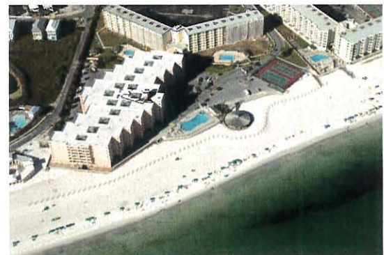
Holiday Isle post-construction conditions
