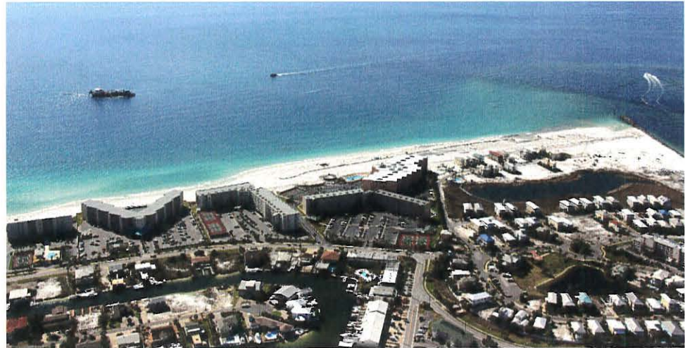
Western Destin Beach Restoration project under construction (February 2013)
