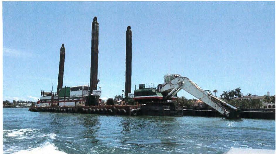
Mechanical dredge on the Intracoastal Waterway
