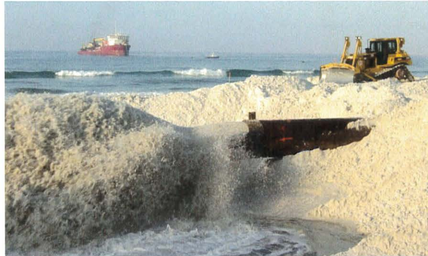
Destin Beach project construction
