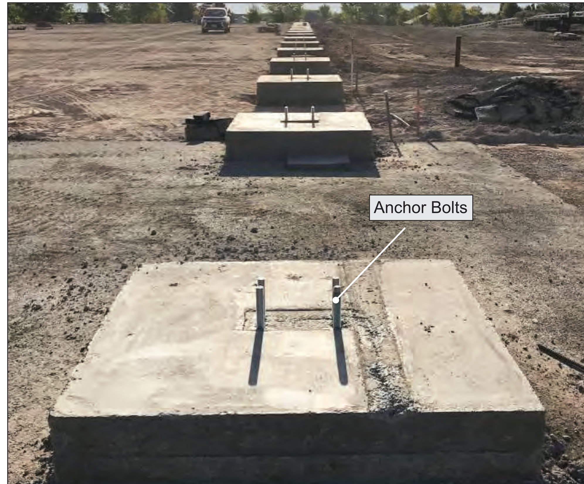
Photo above shows anchor bolts set in concrete. Consult the services of a qualified foundation contractor as needed to install the anchor bolts for your building.
