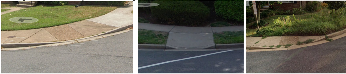
Examples of Older Style ADA ramps
