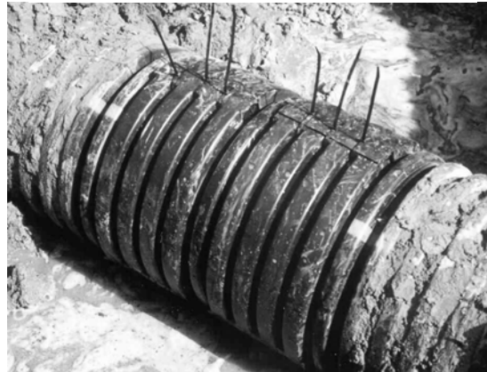
Figure 3 Split Band Installation
