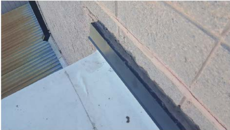
Deteriorated caulk
