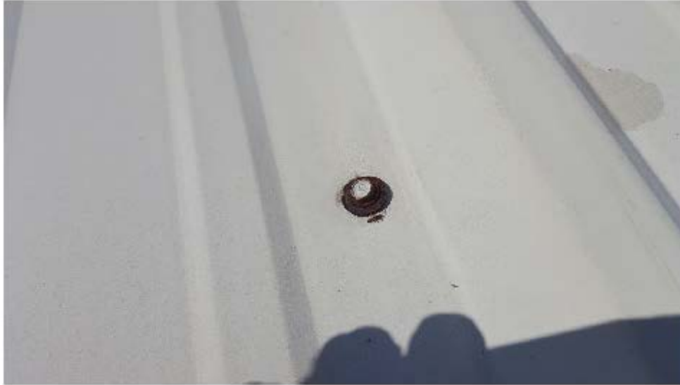
Rusted fasteners
