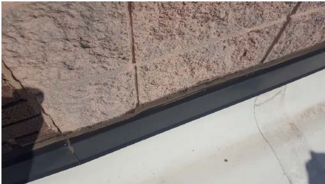
Deteriorating caulk
