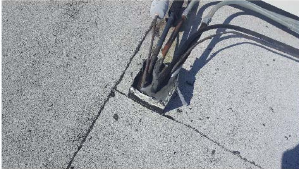
Low pourable sealer in pitch pan
