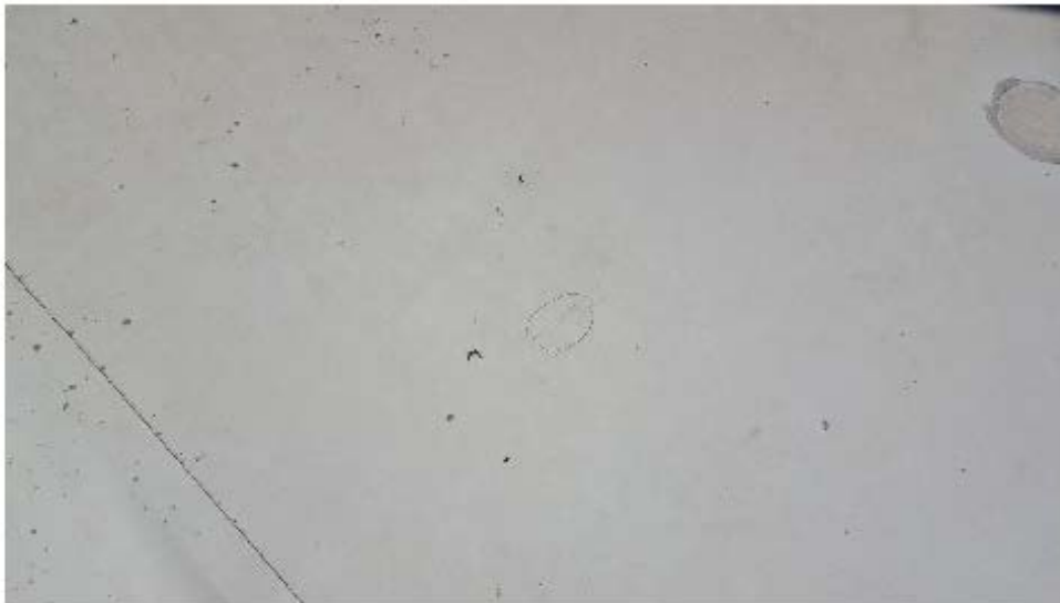
Cut in TPO
