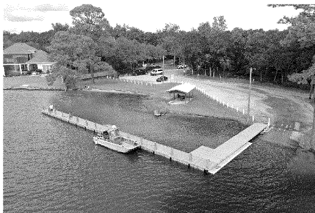
Poquito Bayou Park Wave Fence and Dock Extension
