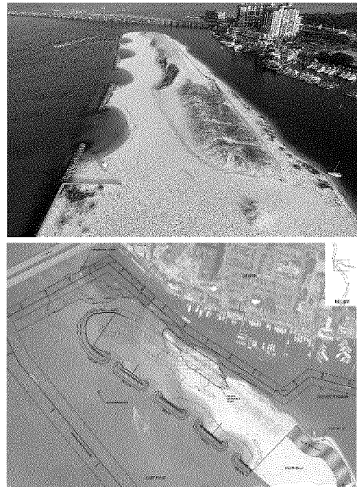
Norriego Point Stabilization Project
