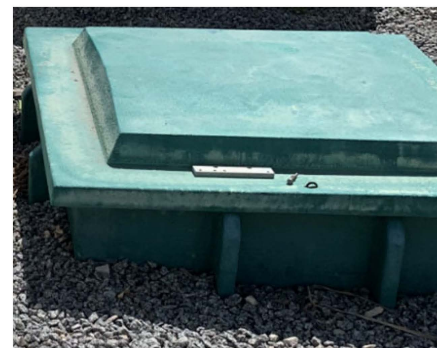
GREEN VAK PAK SURGE TANK
