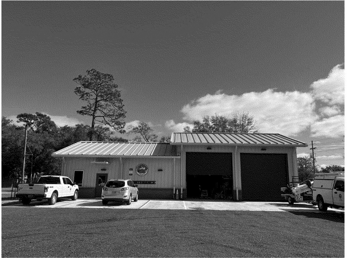
Okaloosa County Water and Sewer Maintenance Building
