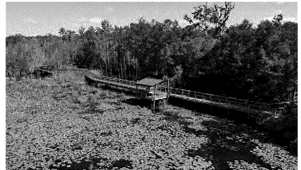
G&A Recently Provided Permitting Services for the SW Greenways & Debbie Lightsey Nature Park Project
