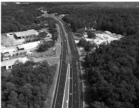
FDOT SR 10 (US 90) Resurfacing in Gadsden County
