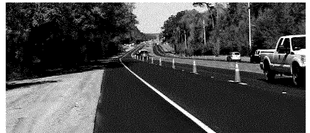
G&A Provides Construction Administration on the Majority of Our Projects
