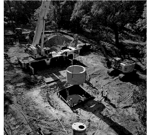
Lake Munson Septic-to-Sewer Conversion Project
