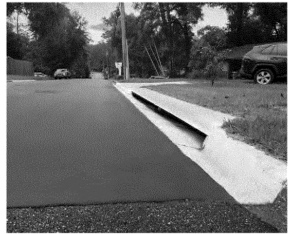
Chestwood Ave Drainage Improvements
