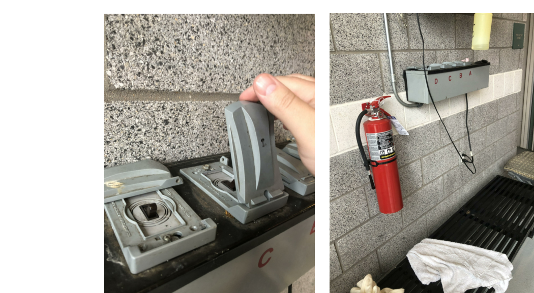
RELOCATE HOSE REEL SOLENOID SWITCH ASSEMBLY
