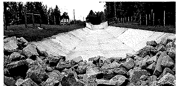
Before (top) and after (bottom) repairs at Alex Reed outfall.
