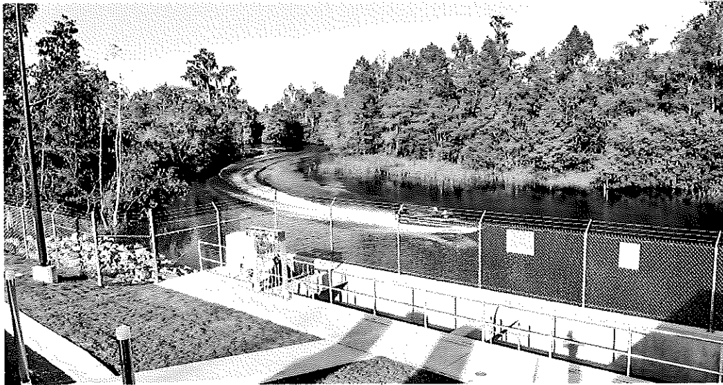
The Alternate Water Supply Project in Bay County pumps raw water from the Deer Point Reservoir to the Water Treatment Plant 11 miles away.
