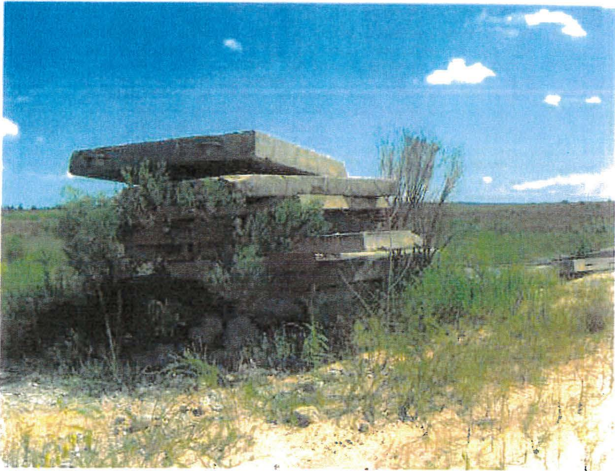
Photo #1 (C-74) Concrete Material
