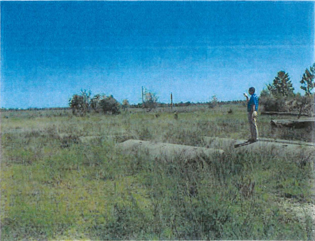
Photo #3 (C-72) Concrete Material
