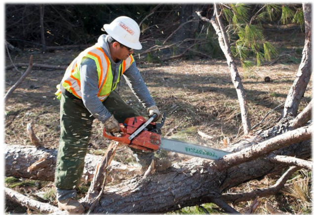
Hazard Tree Removal (Leaner)
