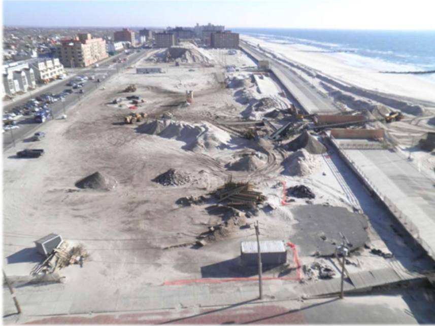
Sand Reclamation and Screening Site
