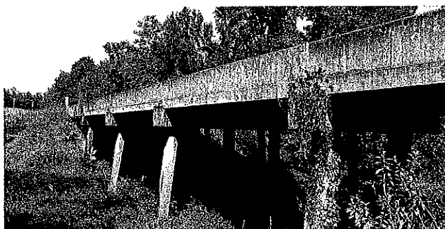
Big Horse Creek Bridge (No. 570085)
